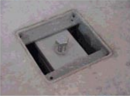
Ready for jacking
